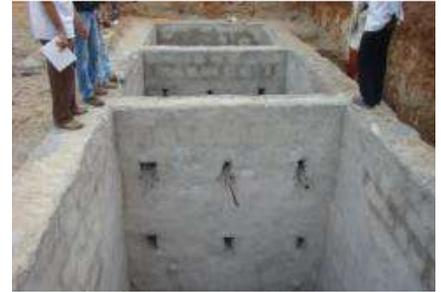
*Underground tanks being prepared for a hotel sewage treatment plant*
