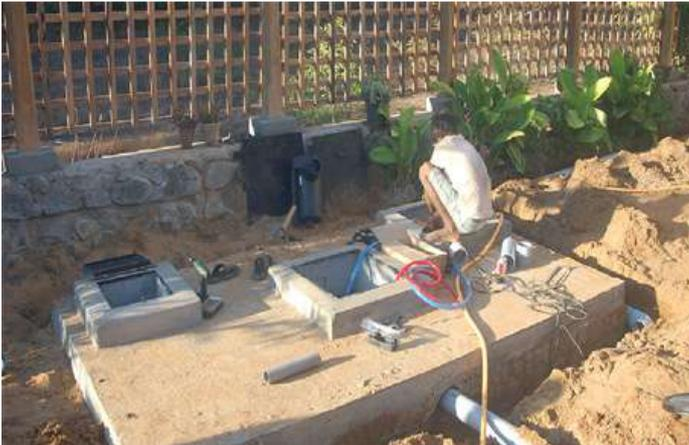
*Single home STP can be installed in hours by local plumber*
